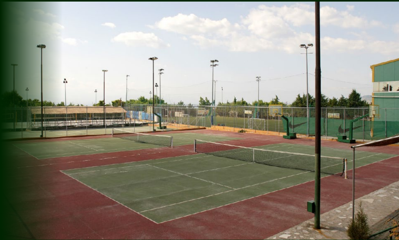
3 tennis courts (Quick surface)
